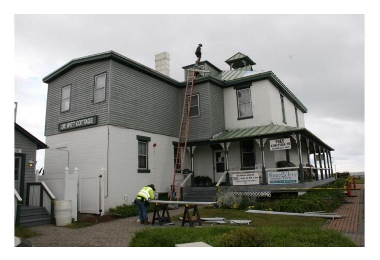
Contractors above are busy applying the new roof on the deWitt Cottage. The new metal roof is made of an alloy that will prevent the roof from rusting like the old roof. The old roof was 30 years old and suffered significant rust damage causing the roof to leak.
